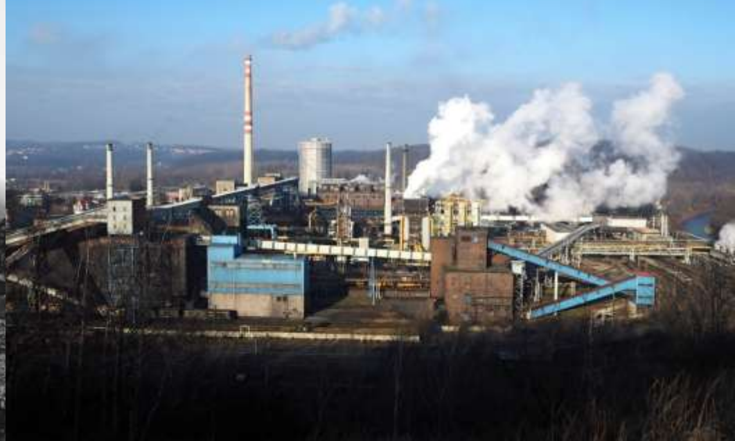
Coke plant in Ostrava, 2021
